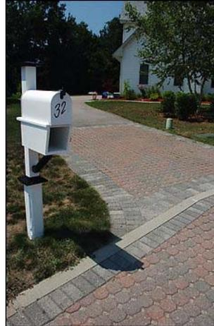
Gaps in permeable concrete pavers draw rainwater into the ground, minimizing runoff. (By Bruce K. Ferguson)
